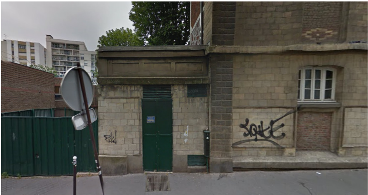
Rue Rampal, Paris
